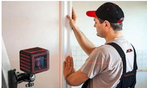
Fig. 5. Wall cladding with a laser level.
