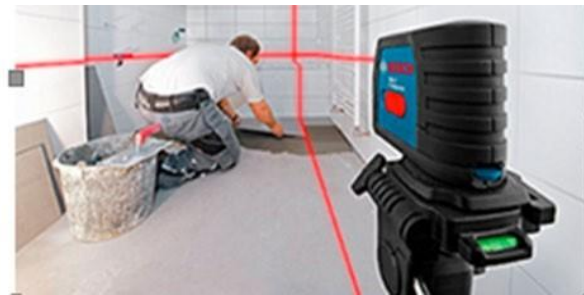
Fig. 6. Floor installation with a laser level.
